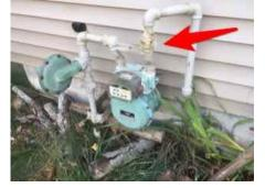
**233:** - The gas meter is outside on the right side of the building. The main gas supply shutoff valve is located on the riser pipe between the ground and the meter. This valve should be turned 90 degrees (either way) in order to shut off the gas.
