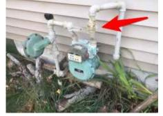
**130:** - The gas meter is outside on the right side of the building. The main gas supply shutoff valve is located on the riser pipe between the ground and the meter. This valve should be turned 90 degrees (either way) in order to shut off the gas.
