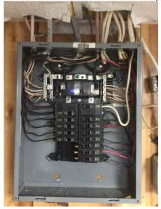
39: - WIRING METHOD: Wiring method: Non-metallic sheathed cable or 'romex'
