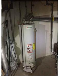
110: - ENERGY SOURCE: Energy source: Natural gas111: - CAPACITY: Capacity: 40 gallons112: - Age: Estimated to be 2 years old
