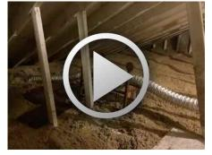
**153:** - The ducts from several bathroom exhaust fans do not go to the exterior. This condition allows excessive moisture to be vented into the attic. We recommend this deficiency be corrected.
